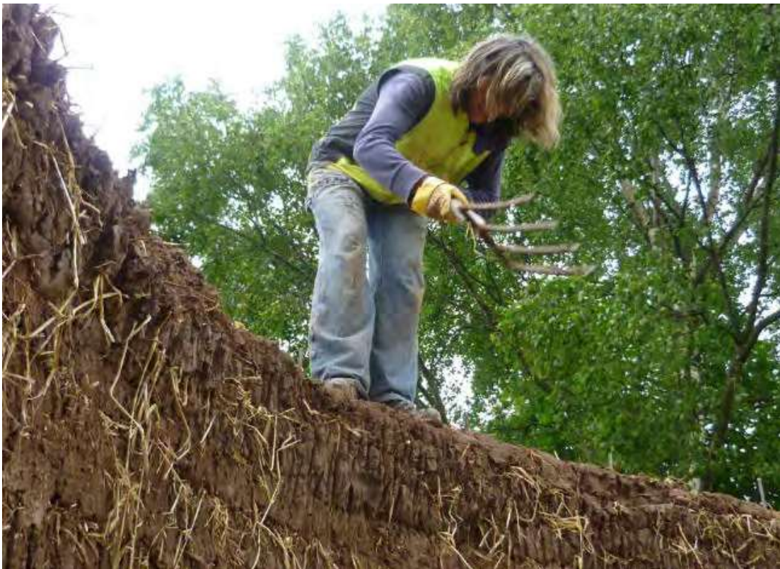
Figure 2: Mudwall being built in the traditional manner.
