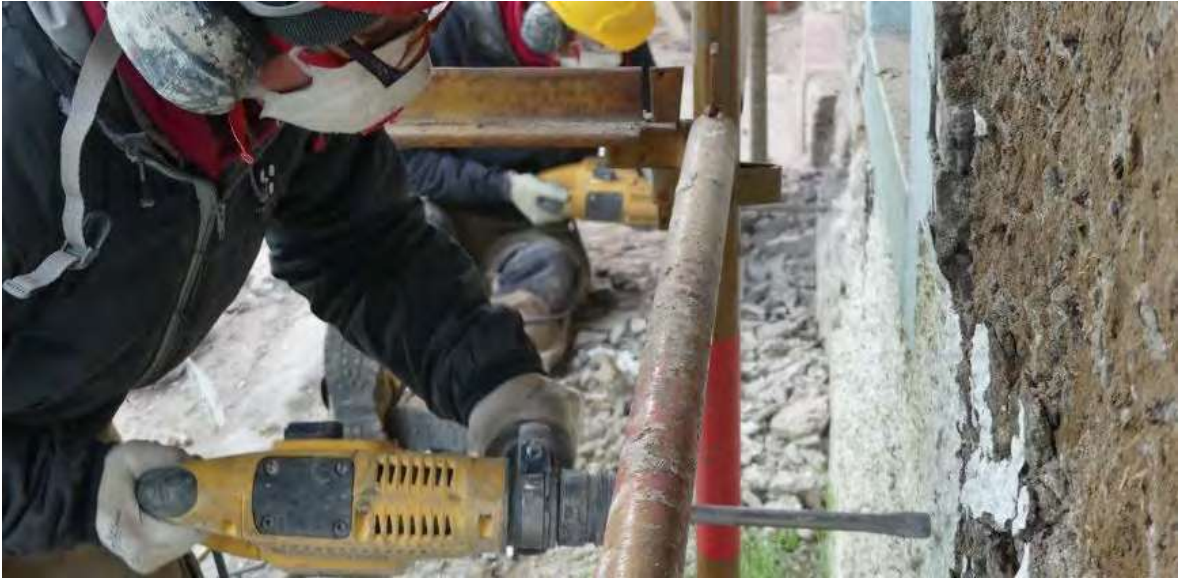
Figure 5: Removing the cement render.
