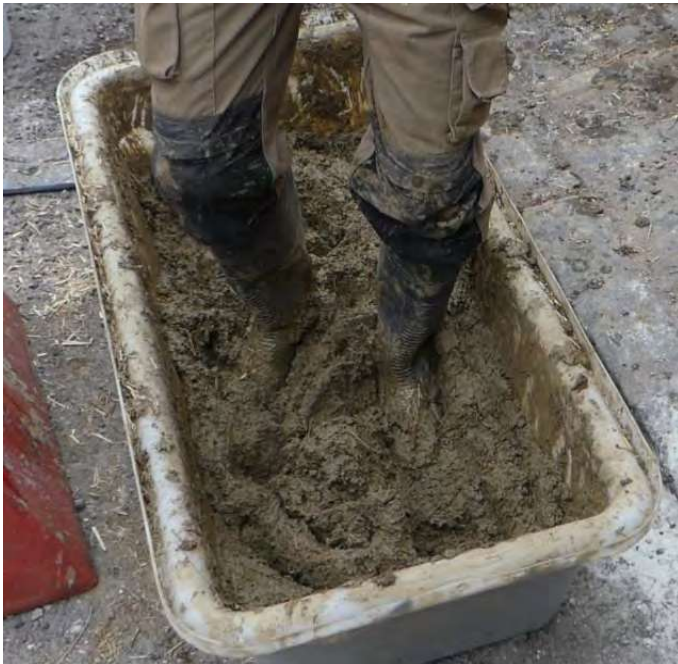
Figure 11: Clay being mixed with sand and straw by foot on site.
