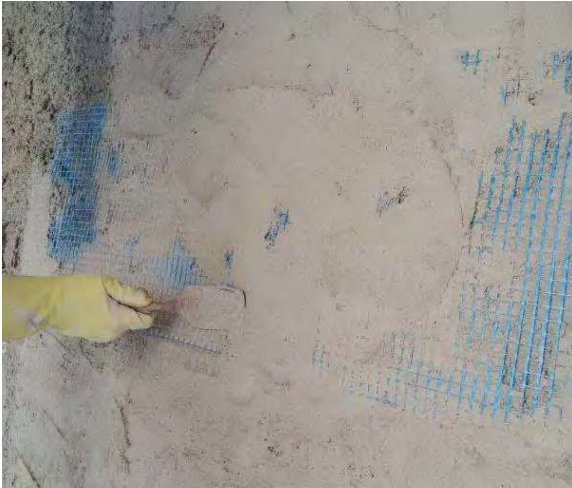
Figure 16: Plastic mesh reinforcement across substrate junctions to prevent cracking of the lime harl.
