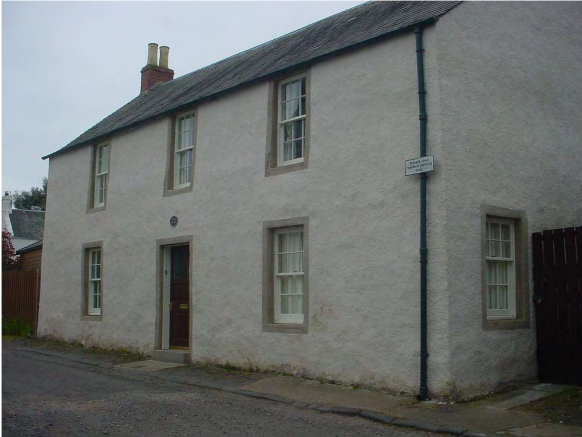
Figure 20: Gray House after the completion of works.
