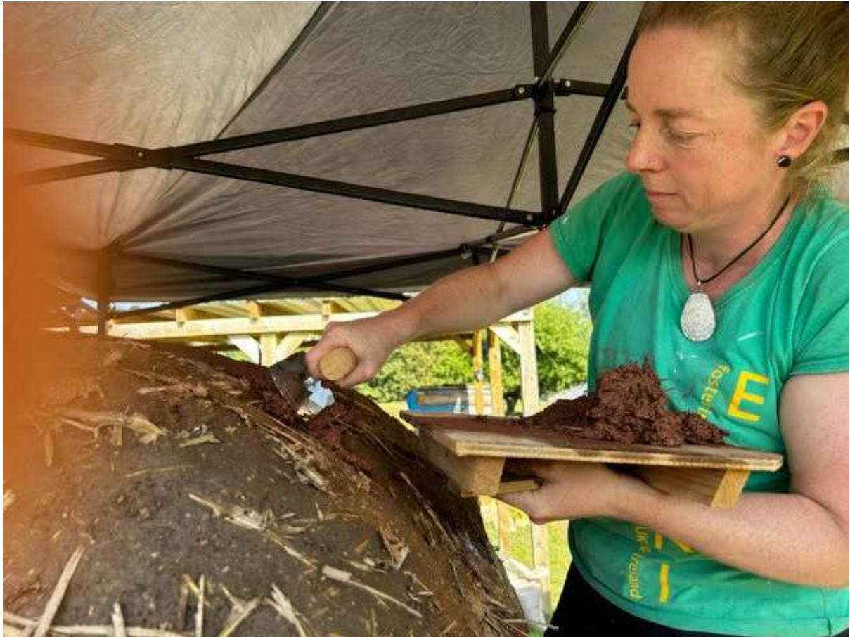
Annabel taught us how to apply the clay to the oven with a flat trowel and how to catch any fallen bits of clay so we wouldn't waste any.
