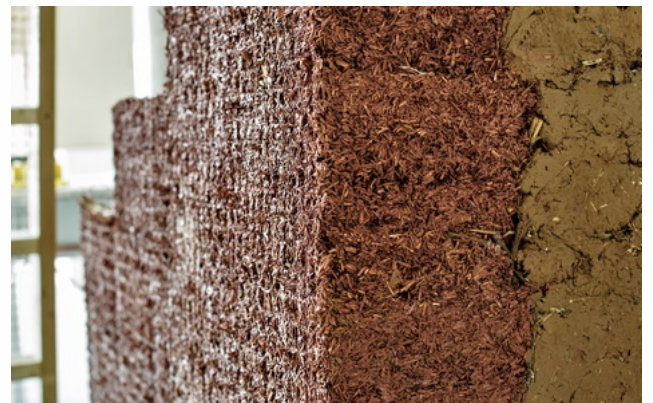
Sample wall showing intersection of cob and light earth mix
